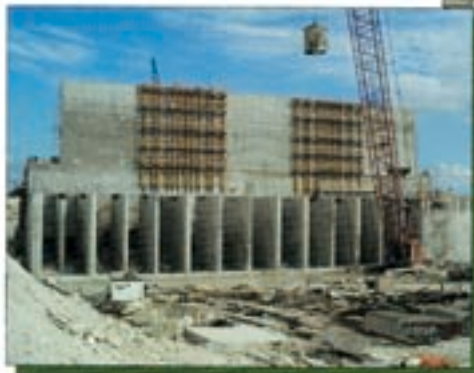
G-335 pump station, intake side of super structure wall
